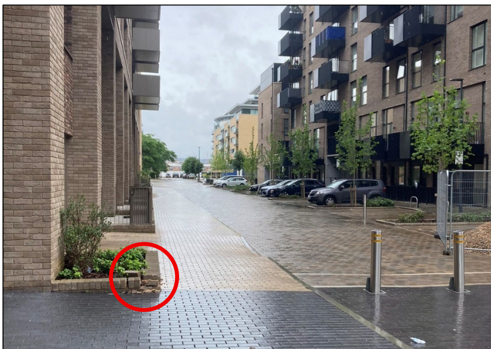
Figure 2 – Site Audit – Damaged Footway on Royal Quay Road
